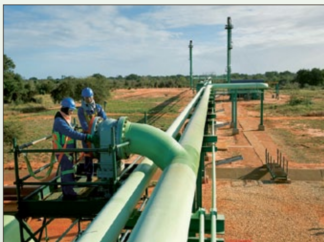
New gas pipeline in Mozambique. The country has invested heavily in energy production for export to neighbouring countries. (Photo Wikicommons)
